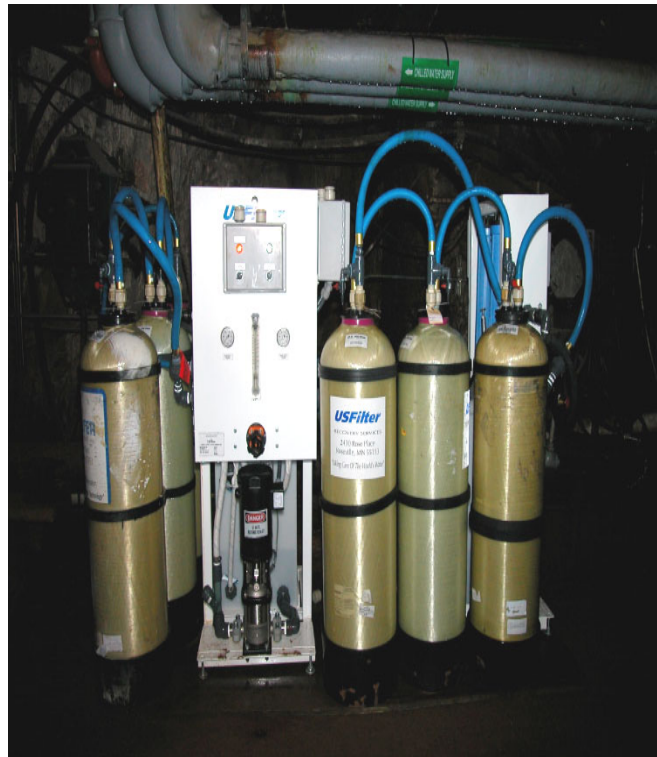
Figure 3-1. In-mine ion exchange treatment, Soudan Mine. (3.7 ft 3 tanks)
