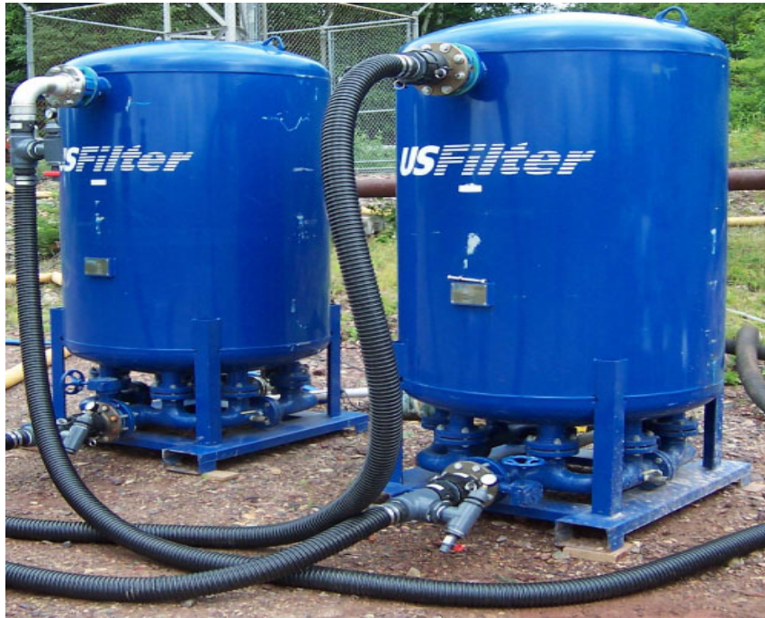
Figure 3-2. Ion exchange resin tanks (60 ft 3 ), Soudan Mine.
