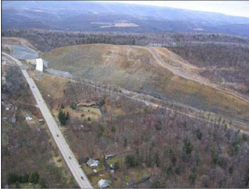
Figure 1-1. Aerial view of the Skytop cut on January 6, 2005 looking north. Existing Route 322 in foreground. Future I-99 roadbed runs along the base of the cut. Black plastic covers one of several areas of pyritic fill as a stopgap measure to minimize water infiltration. (Photograph courtesy Keith Brady)
