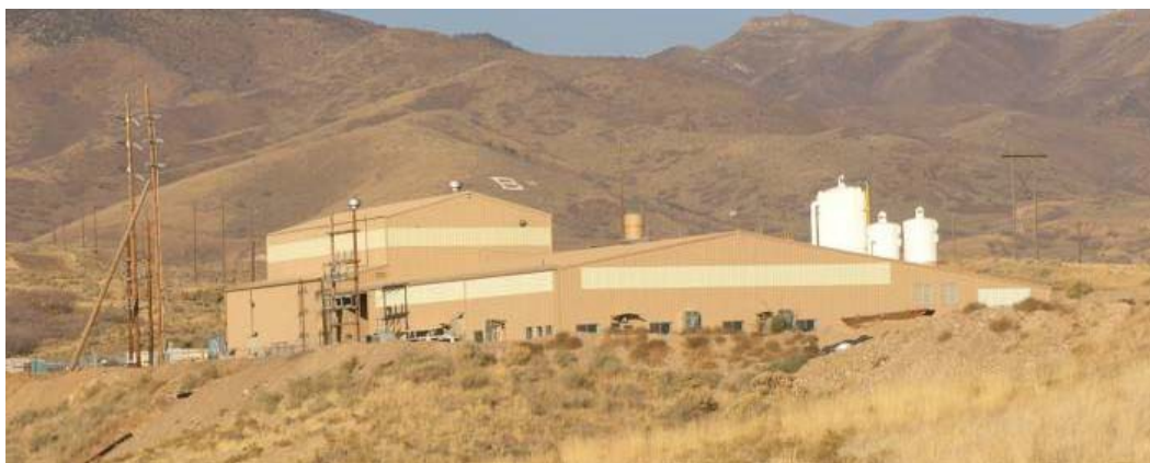
Figure 2-2. The Bingham Canyon Water Treatment Plant. (The overall facility site is 2.5 acres; the BCWTP itself is 14,600 square feet.)
