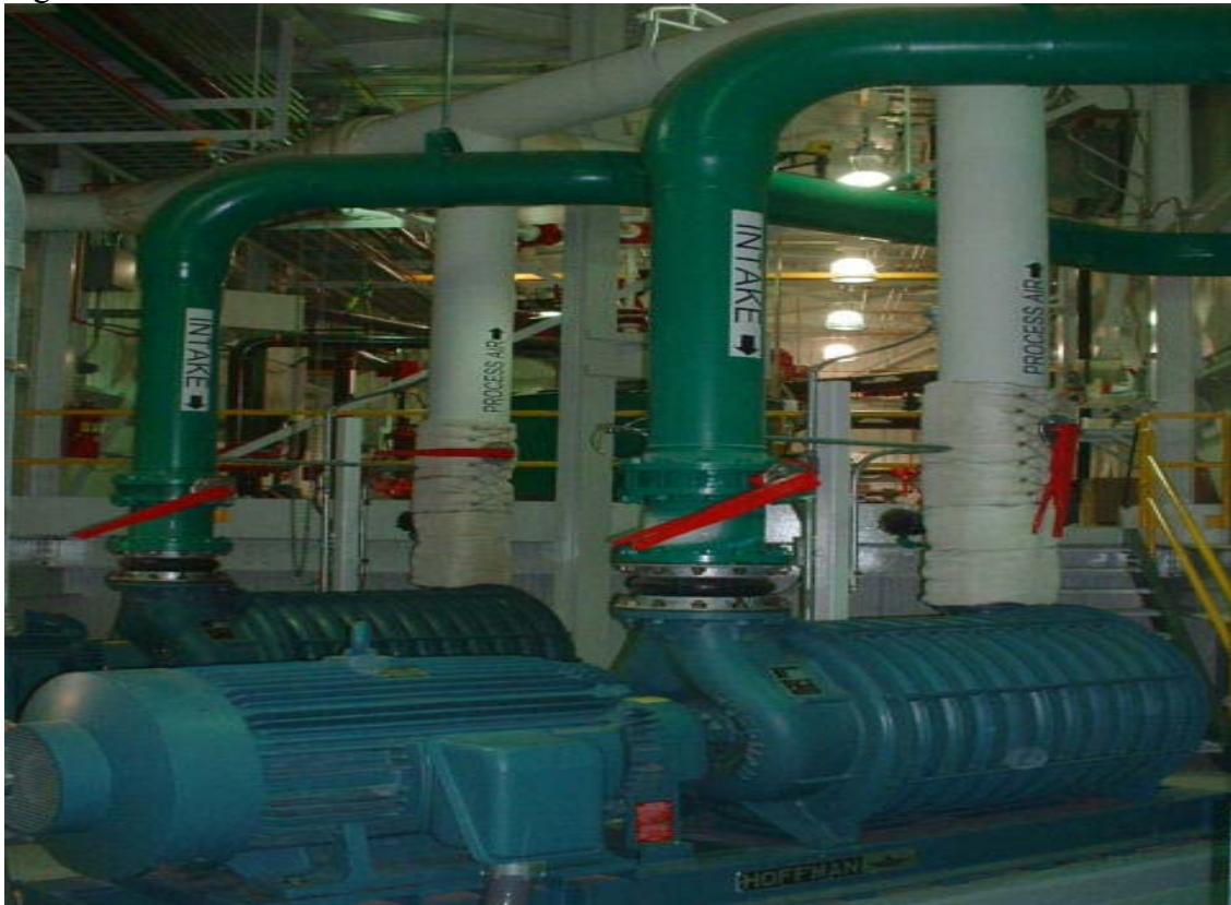
Figure 12. Blower Installation
