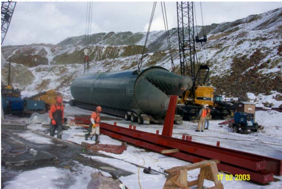
Figure 5. Lime Silo Pre-lift
