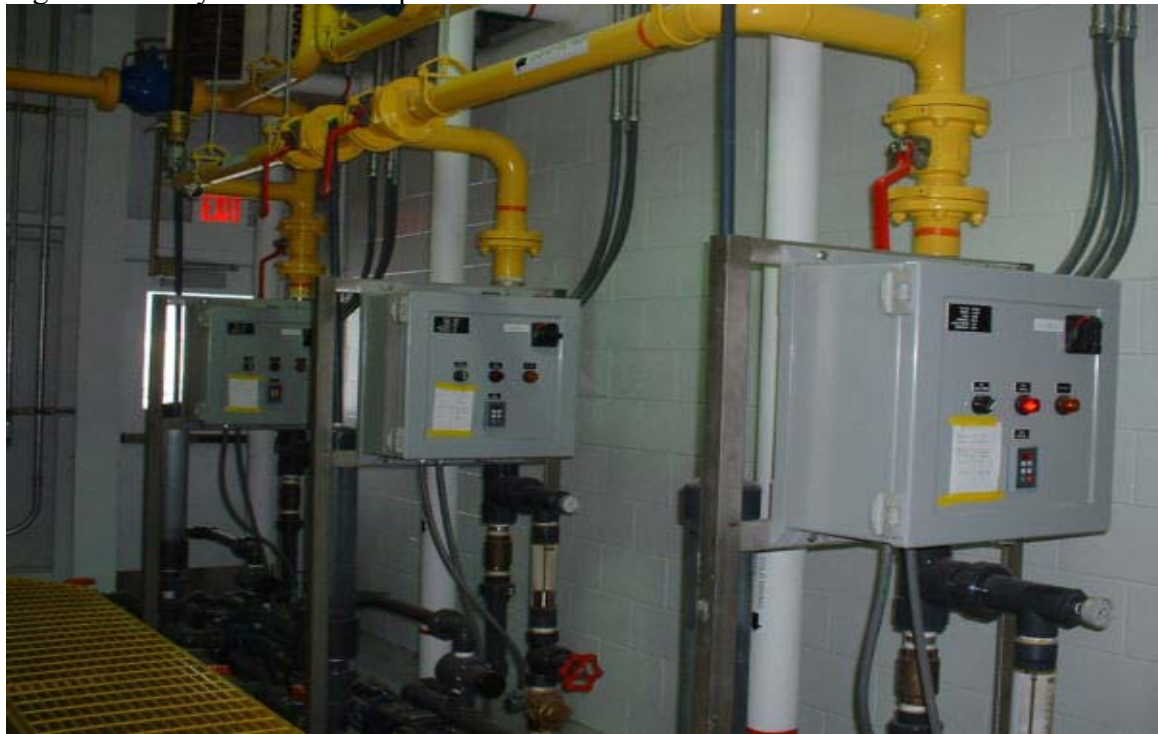
Figure 17. Polymer Feed Pumps and Controls
