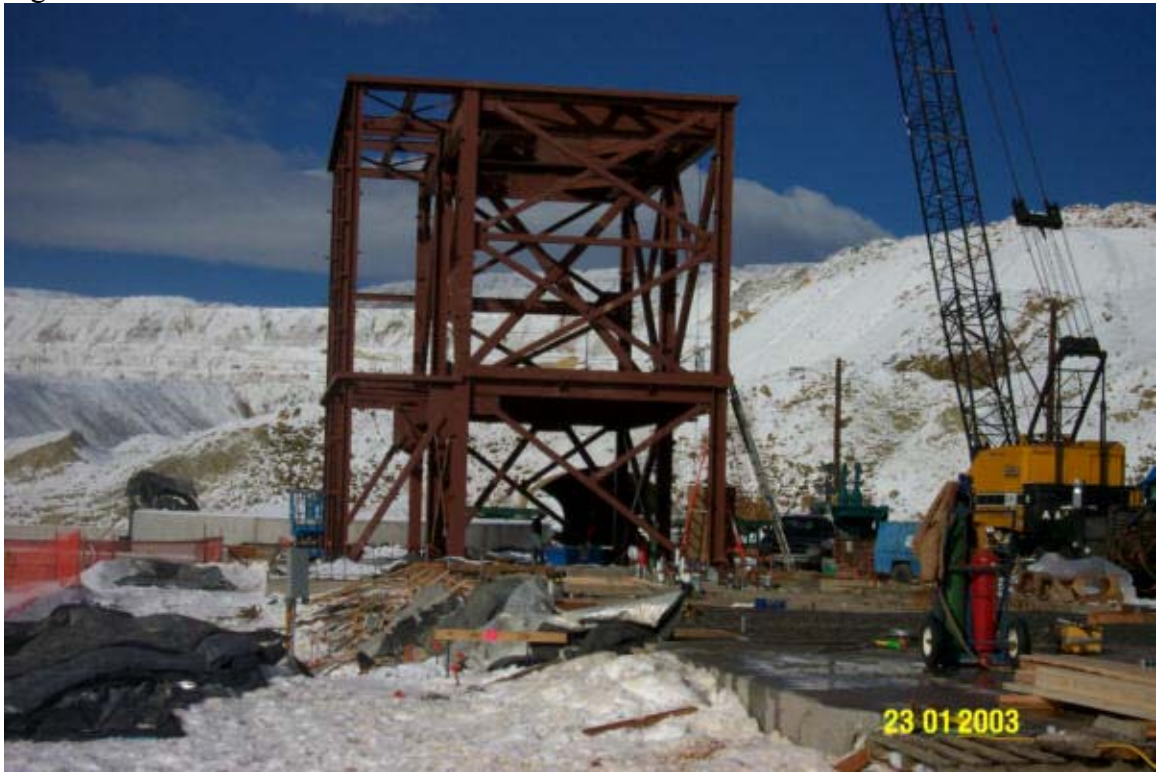
Figure 5. Lime Silo Pre-lift
