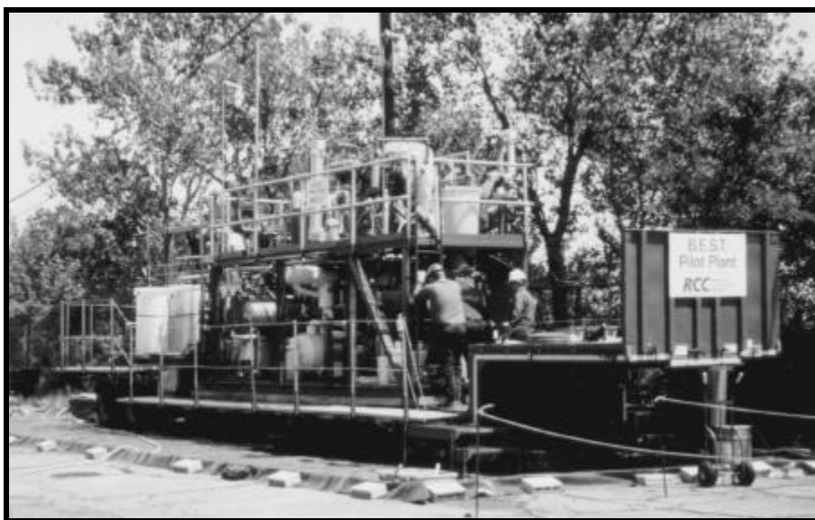
Example of a Contaminated Sediment Remediation Project Using BEST Equipment
