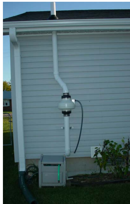
Figure 4-3. Active subslab depressurization system.
